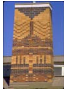
Detail of chimney
