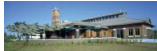
Panoramic of Frederiksen Court Community Center.
