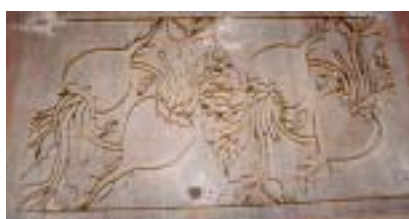
Beets outlined in brass before the terrazzo installation.
